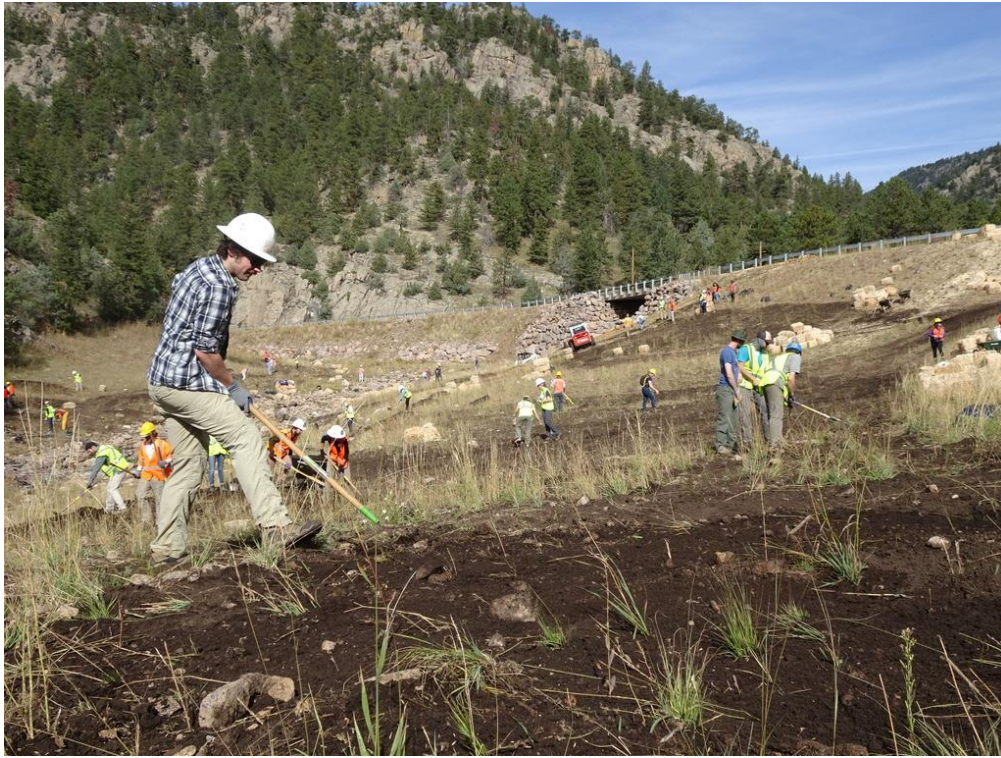
Restoration area on 9/30/2017: riparian zone up to highway, Big Elk Road in background. Note topsoil dressing on parts of the restoration. Erosion matting used on steep slope below road. Following spreading of topsoil, seeding, raking, and woodstraw applied.
