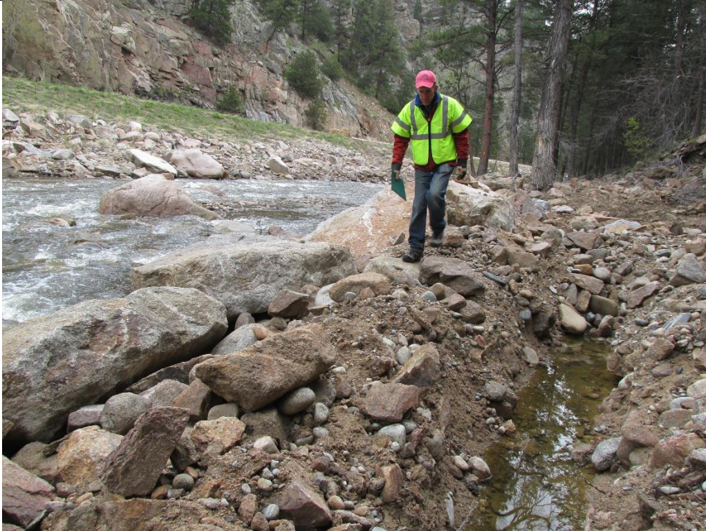
April 30, 2016, view down stream of willow trench post-construction. Note groundwater in trench bottom.
