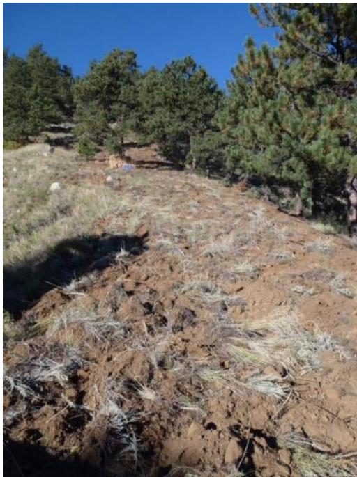
Looking west at the lower portion of the road obliteration project area after road obliteration by heavy equipment. The site is ready for seeding and scattering of coarse woody debris. Barring excessive human traffic, the restoration would most likely have been successful. October 2014.
