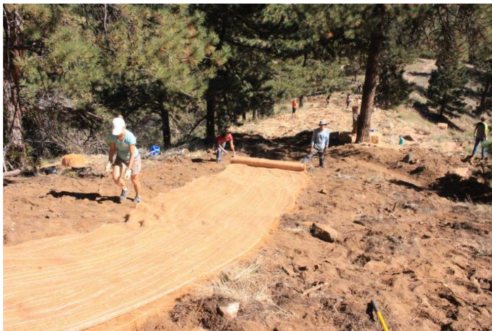
Looking east near the middle of the project area at erosion mat being installed on a particularly steep slope. Project day, October 4, 2016
