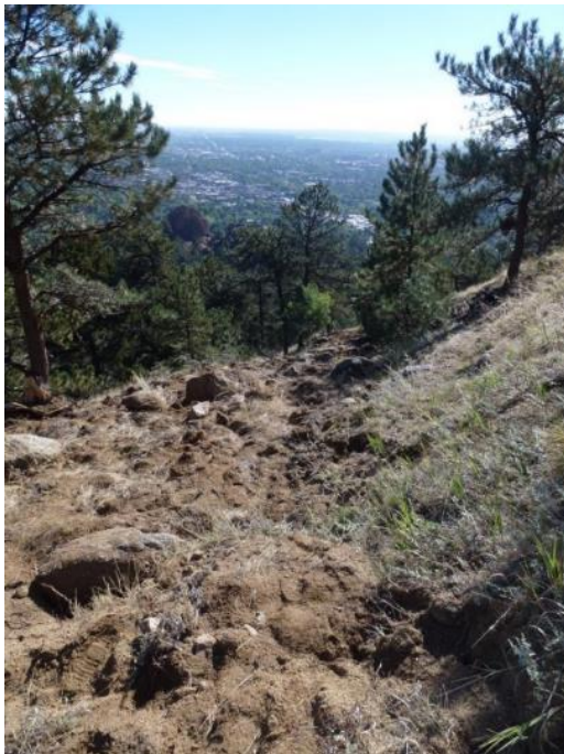
Looking east at the middle portion of the road obliteration project area after road obliteration by heavy equipment. The site is ready for seeding and scattering of coarse woody debris. Barring excessive human traffic, the restoration would most likely have been successful. October 2014.
