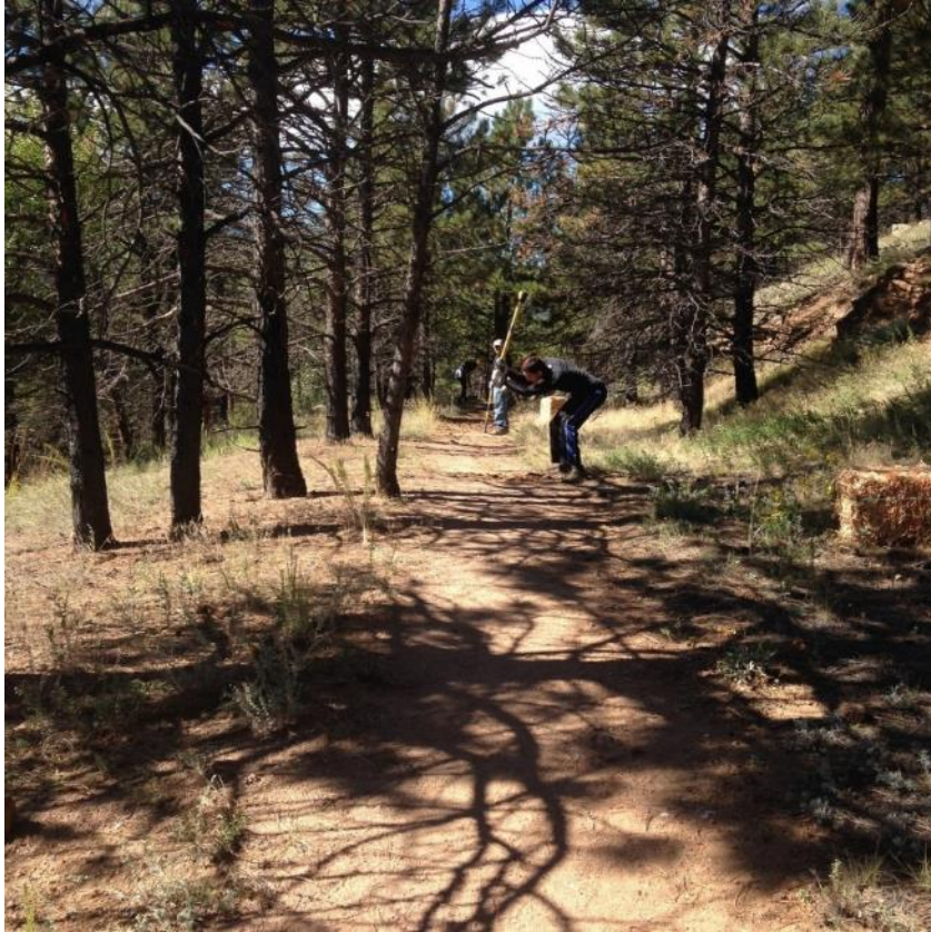
Looking west at a segment of level trail being scarified prior to seeding and application of wood staw.
