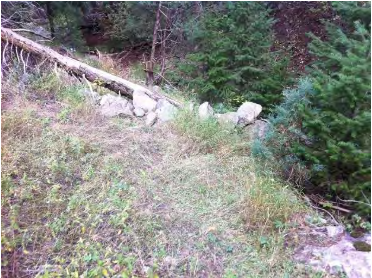
Section E, very nice water bar made with a combination rock and log, holding well, allowing vegetation to build up on the uphill side.
