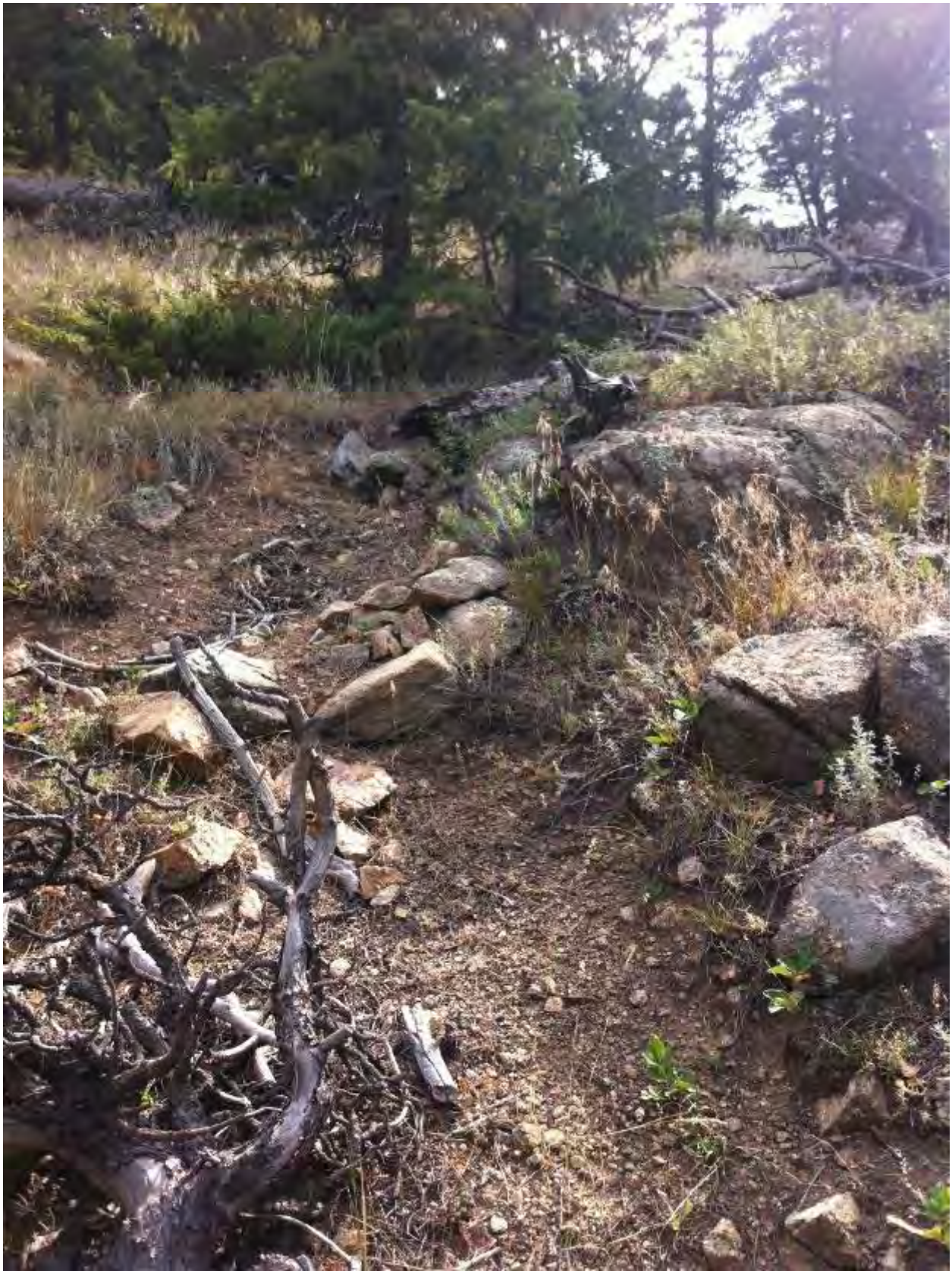
Water bar along Section A, which is holding well.
