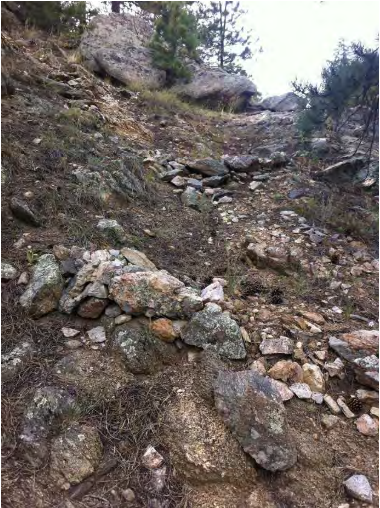
Very steep section of Section A, with water bars holding very well, trail has lots of sediment deposition on top of it.
